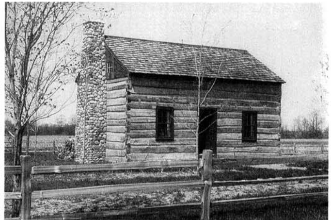
Reconstructed log home at the site of the Peter Whitmer, Sr., home in Fayette, New York. Here the Book of Mormon translation was completed, the testimony of the Three Witnesses was signed (June, 1829), and the Church was organized on April 6, 1830. Twenty revelations in the Doctrine and Covenants were received here. Courtesy LaMar C. Berrett.
